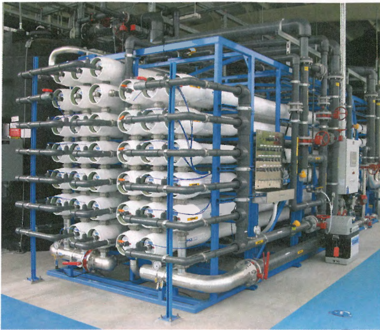
REVERSE OSMOSIS , done in long white cylinders ( above left ), removes salts and microscopic impurities from one million gallons of wastewater a day at the San Diego Advanced Water Purification Facility. The final product is almost as pure as distilled water.
